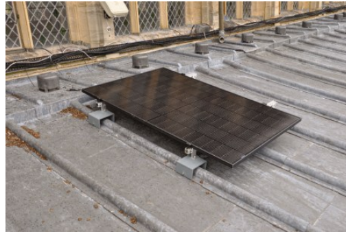
Trial solar panel on the South aisle roof
